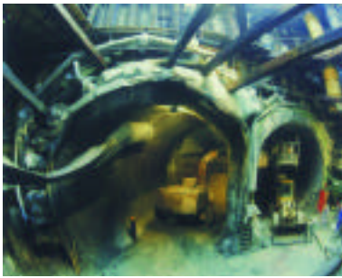
Constructing a traffic tunnel by using the sequential excavation method
