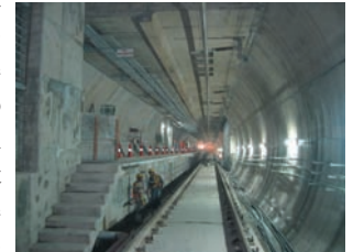
Delhi Metro station
