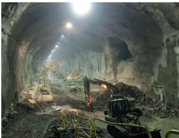
Figure 60 : 72 nd Street Station Cavern during drill and blast excavation and initial support phase, Second Avenue Subway, New York City. (Photo Brian Fulcher).
