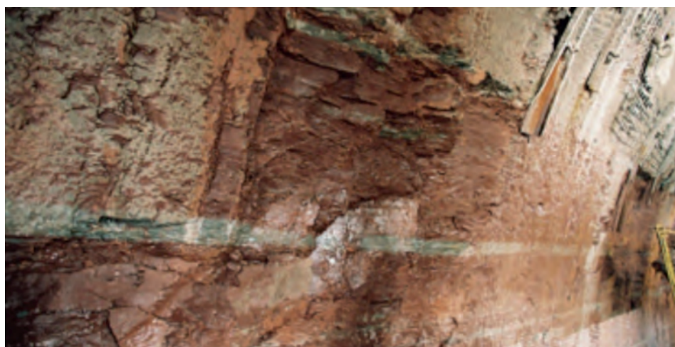
Figure 23 : Niagara Tunnel Project – Rock Conditions. View of freshly cut tunnel wall showing the degradation, strata and high clay content. (photo from B. Fulcher).
