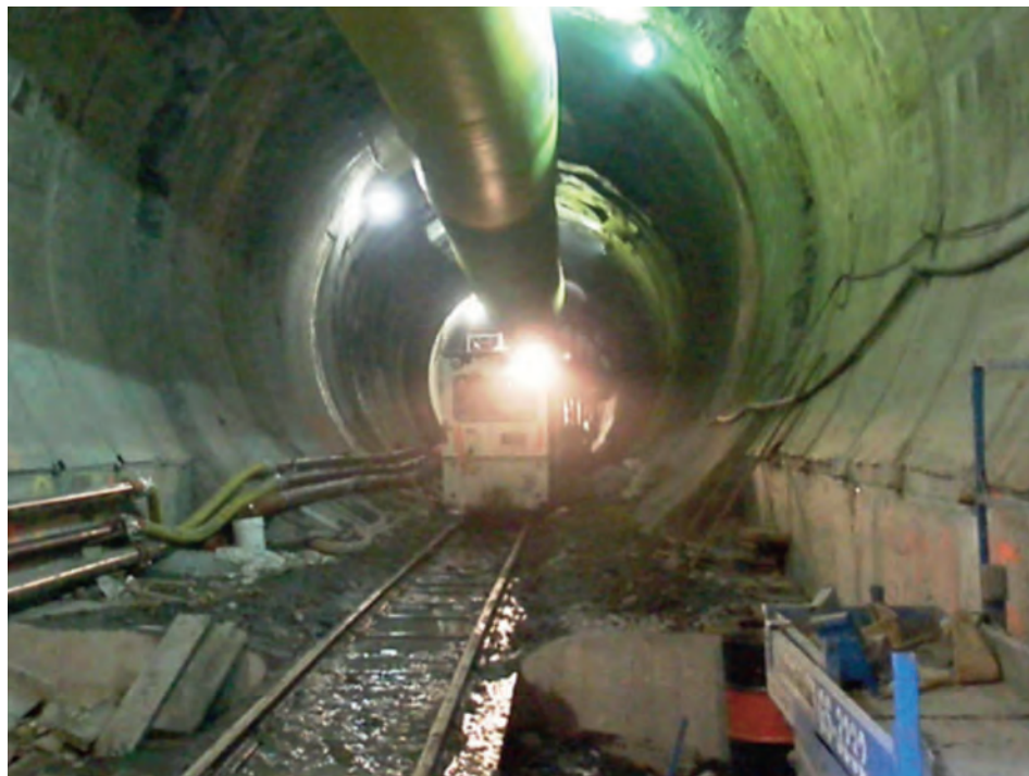
Figure 62 : Rail transport in tunnel.
