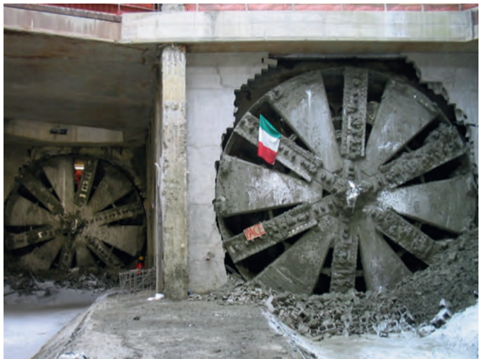
Figure 52 : Break-through of two EPB machines at the Bologna railway junction, Italy.
