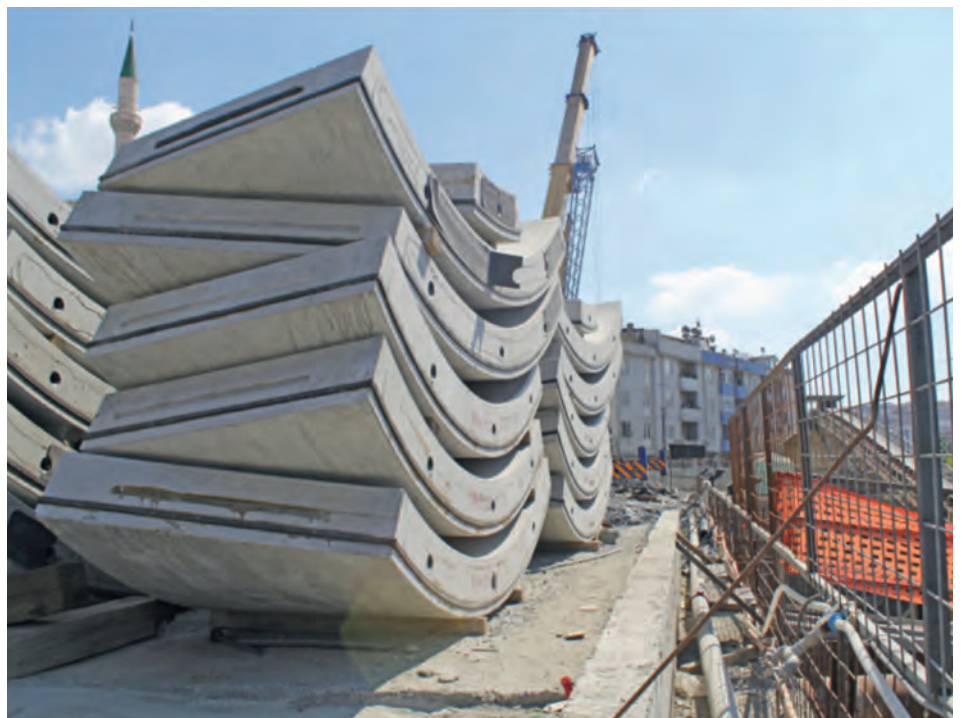
Figure 11 : High strength precast concrete tunnel lining segments.
