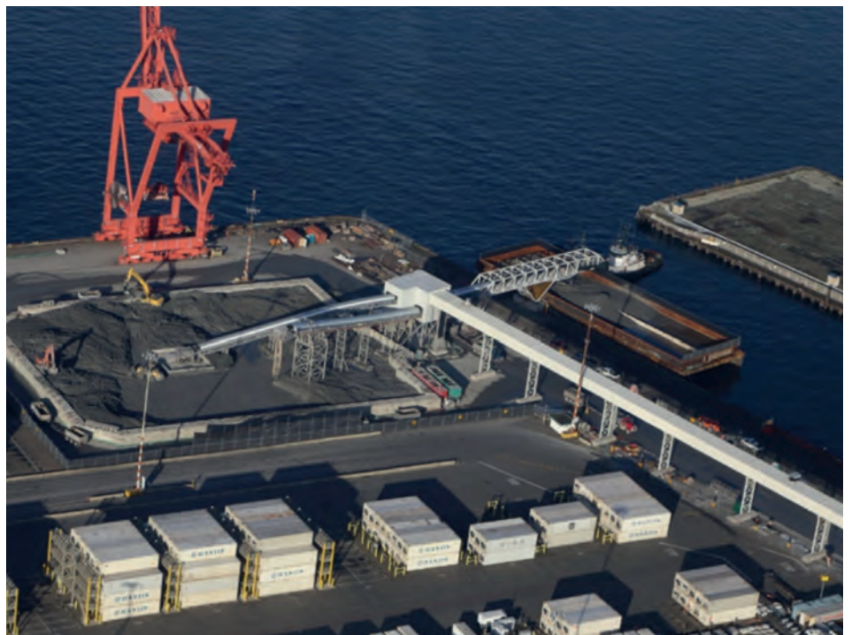
Figure 57: Muck handling and barge loading for the SR 99 project in the harbor of Seattle, Washington, USA.
