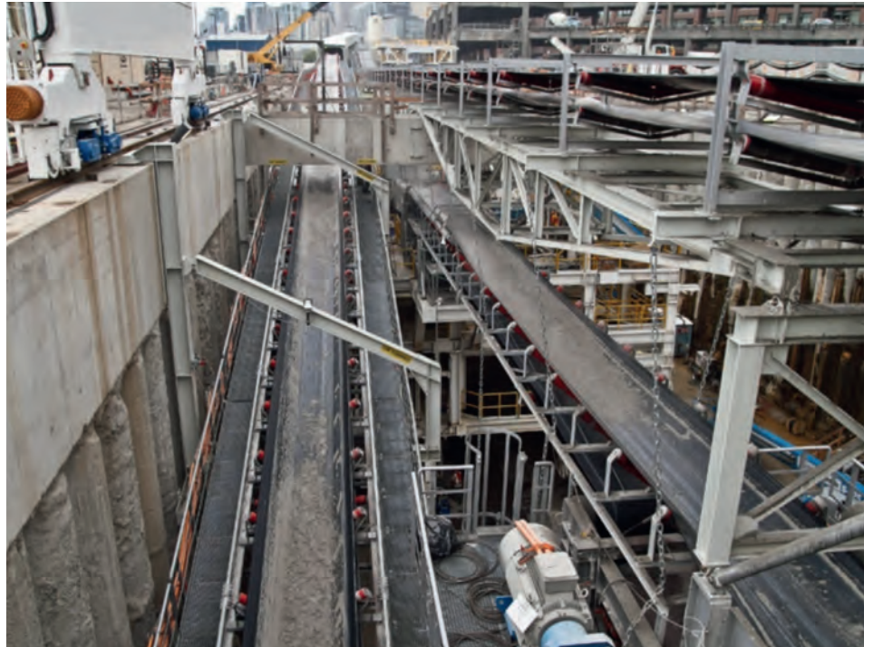
Figure 56 : Conveyor belt transport system at the SR 99 Tunnel in Seattle, Washington, USA.
