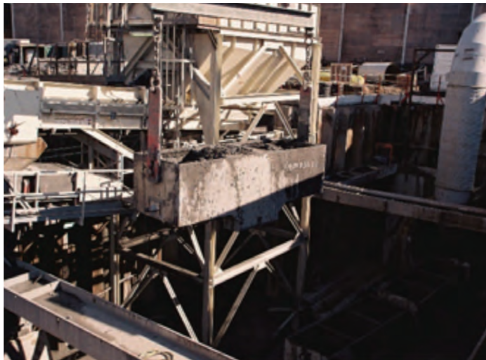
Figure 41: Brightwater Sewer Tunnel, Seattle, USA Tunnel muck (EPB TBM) from shaft for conveyance to marine disposal site. (photo from B. Fulcher).
