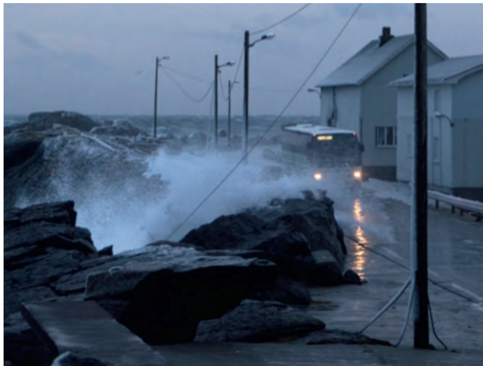
Figure 14 : From Lofoten, Norway, with heavy storms from the Norwegian sea. Large boulders from blasted rock are used as wave breakers in subsea embankment up to 3m below sea level along the shore for erosion protection.
