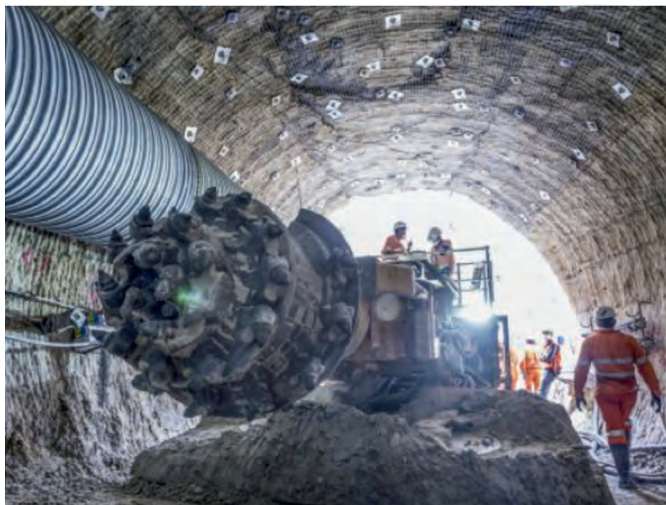
Figure 47: Roadheader used in soft rock (site unknown).
