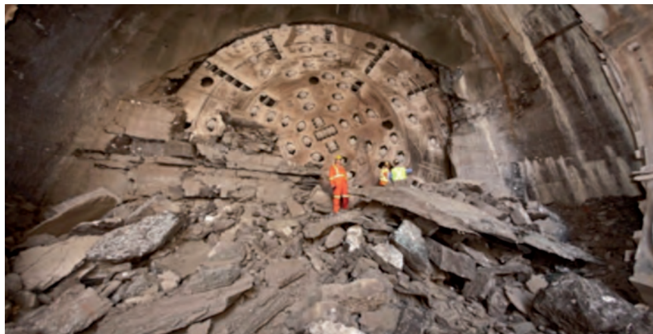
Figure 22 : Break-through of TBM (Robbins) at the Niagara Tunnel Project, Niagara Falls, Ontario, Canada. (photo from Robbins).
