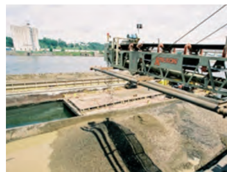
Figure 30 : Portland West Side Combined Sewer Tunnel muck (slurry TBM) loaded on barge for marine site disposal. (photo from B. Fulcher).
