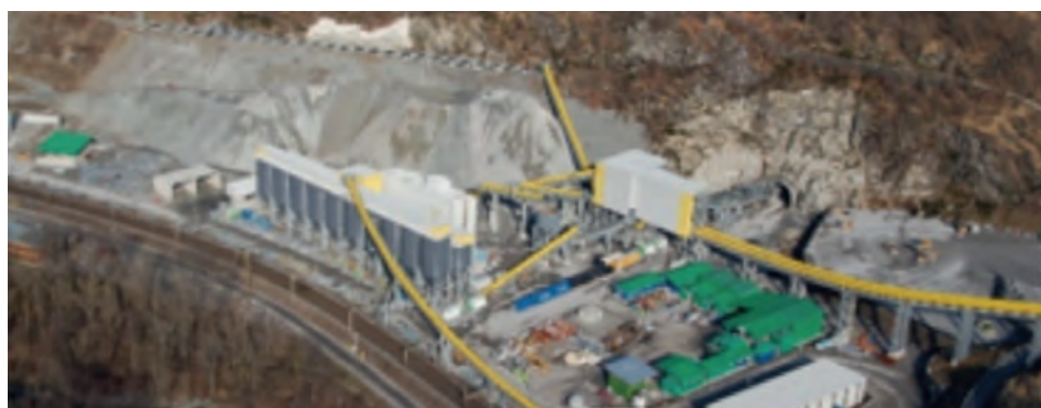
Figures 1 and 2 : Left - Tunnel muck is a valuable resource (photo Ø.Fæhn, Skanska Norge AS). Right - Material depot and gravel plant for the aggregate production in Sigirino (photo Ø AlpTransit Ceneri)
