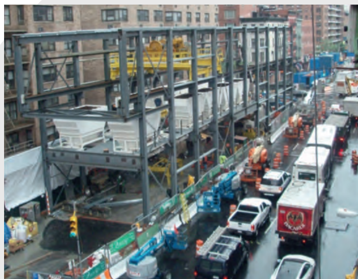
Figure 61 : 72 nd Street Station Cavern spoil handling facility at street level during drill and blast excavation and initial support phase, Second Avenue Subway, New York City. (Photo Brian Fulcher).
