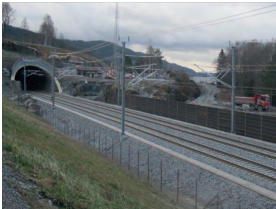
Figure 40 : Railway ballast from crushed crystalline rock. The Joint Venture Rail/Road Project Dovrebanen/E6 Highway along Lake Mjøsa, Norway (photo Sjur Krogstie).
