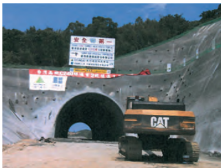
Figure 48 : Soft rock tunneling, the Taiwan High Speed Rail, excavated by backhoe excavators and no explosives used (Rohde 2002).
