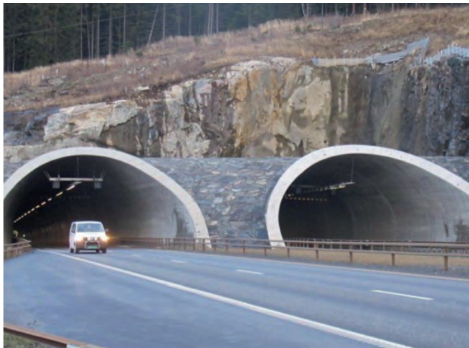
Figure 39 : Aggregates from crystalline rock used in road pavement and fill/masonry/rip rap around portals. The Joint Venture Rail/Road Project Dovrebanen/E6 Highway along Lake Mjøsa, Norway. (photo Sjur Krogstie).
