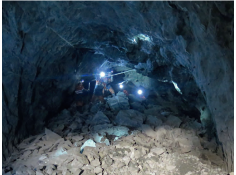
Figure 51 : Drill and blast muck pile from the Rosten HEPP (Photo Ø. Fæhn, Skanska).
