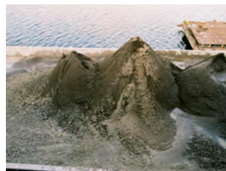
Figure 30 : Portland West Side Combined Sewer Tunnel muck (slurry TBM) loaded on barge for marine site disposal. (photo from B. Fulcher).
