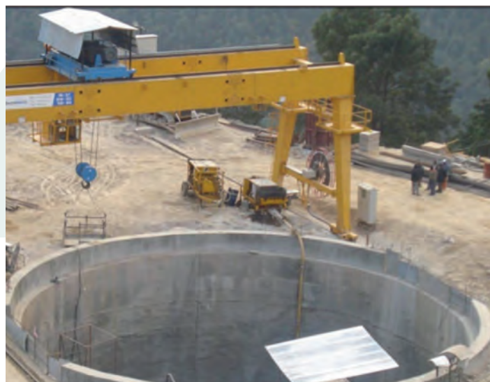
Figure 59 : Hauling of tunnel muck via vertical shaft by crane. (site unknown).
