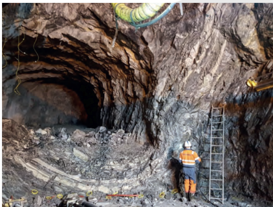
Figure 50 : Charging at the OREA Sewer Plant Extension, Norway. (Photo E. Hannestad, Sweco Norge AS).
