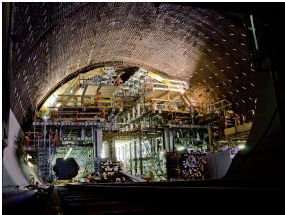
Figure 84 : Concrete made with aggregates from TBM muck, lane change in Faido (photo AlpTransit Gotthard)
