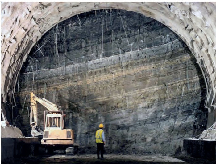
Figure 18: ADECO-RS method applied in the Tartaguille Tunnel. TGV Lyon-Marseilles (France).
