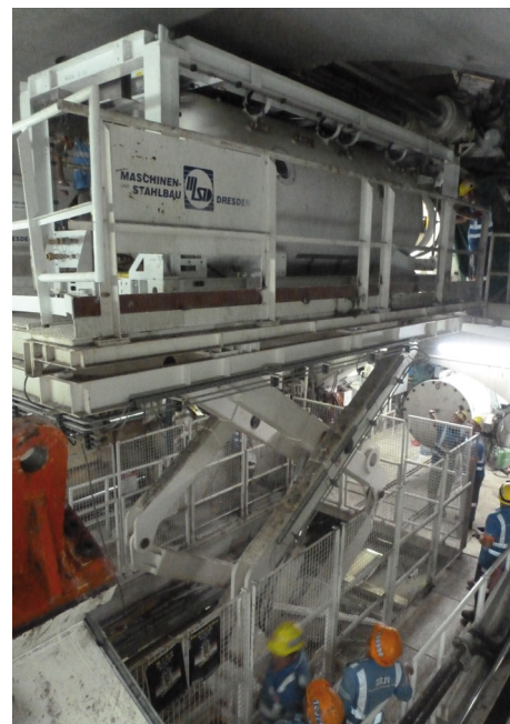
Figure 2 : TUP shuttle being mated to TBM lock
