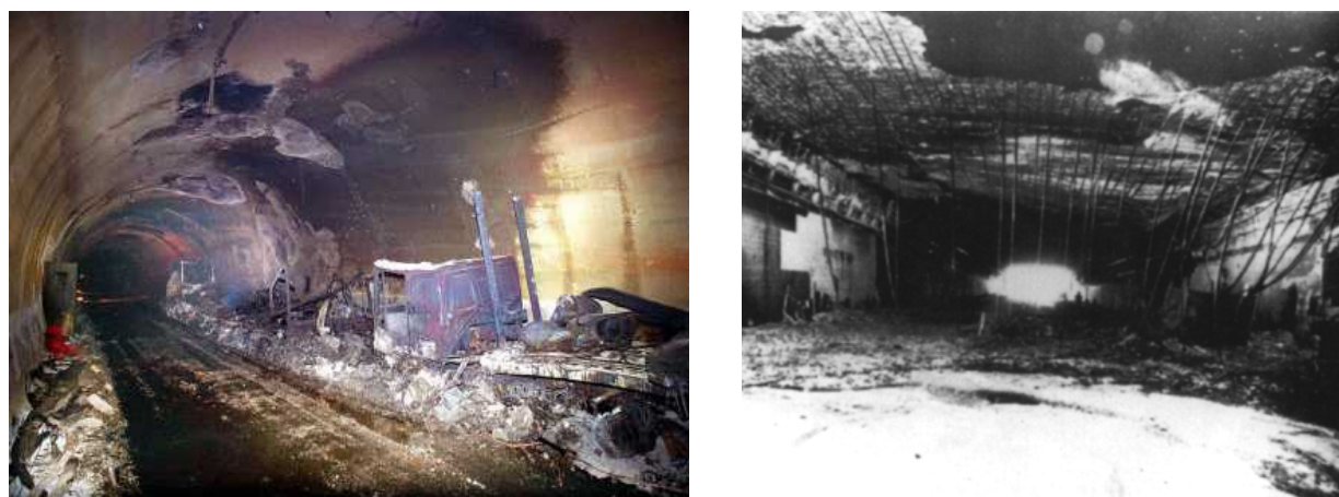
Figure 3.2 Structural damage to tunnels. To the left is shown the damage of the lining of the Mont Blanc Tunnel after the 1999 fire. To the right the severe spalling and detachment of the reinforcement after the fire in the Moorfleet Tunnel in 1968.
