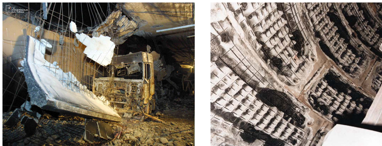
Figure 3.1 Fire damage to the tunnel structure. To the left: the local collapse of the ceiling after the fire in the Gotthard tunnel in 2001. To the right: the severe spalling of the segmental lining after the fire in 1996.
