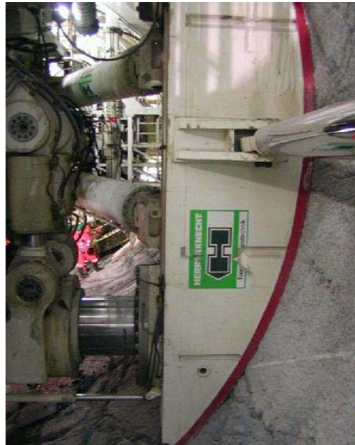
Fig. 4: Tunnel excavation for the Gotthard Base Tunnel, Switzerland, section Bodio-Faido, using a TBM
