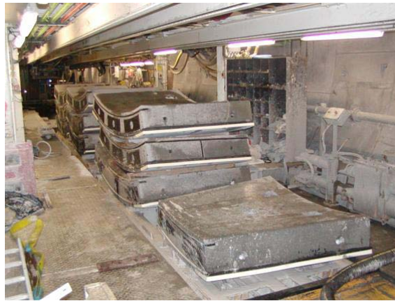
Fig. 5: Crossing the river Thames by the high speed railway line between the Euro Tunnel and London applying a segmental lining made of fireproof concrete
