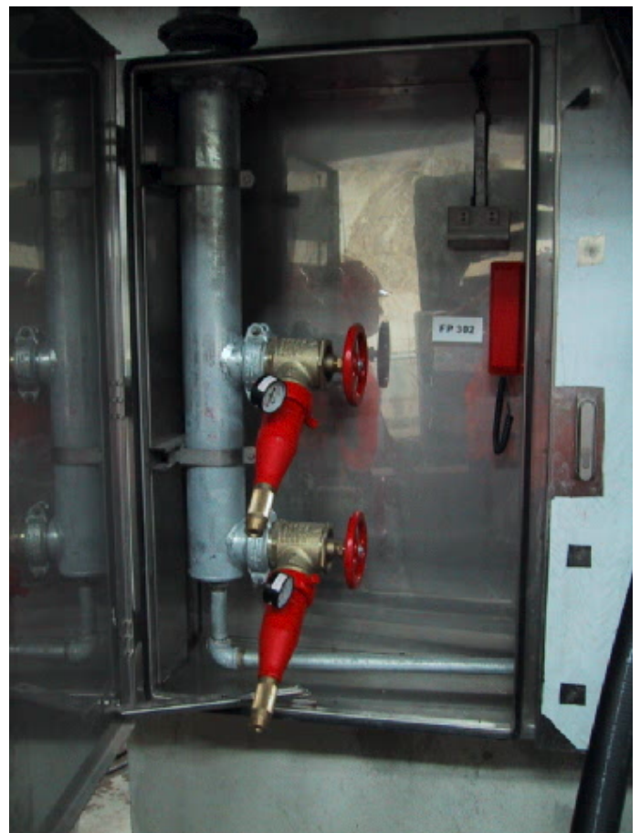
Figure 3 Fire Hydrant and Pressure Testing Equipment
