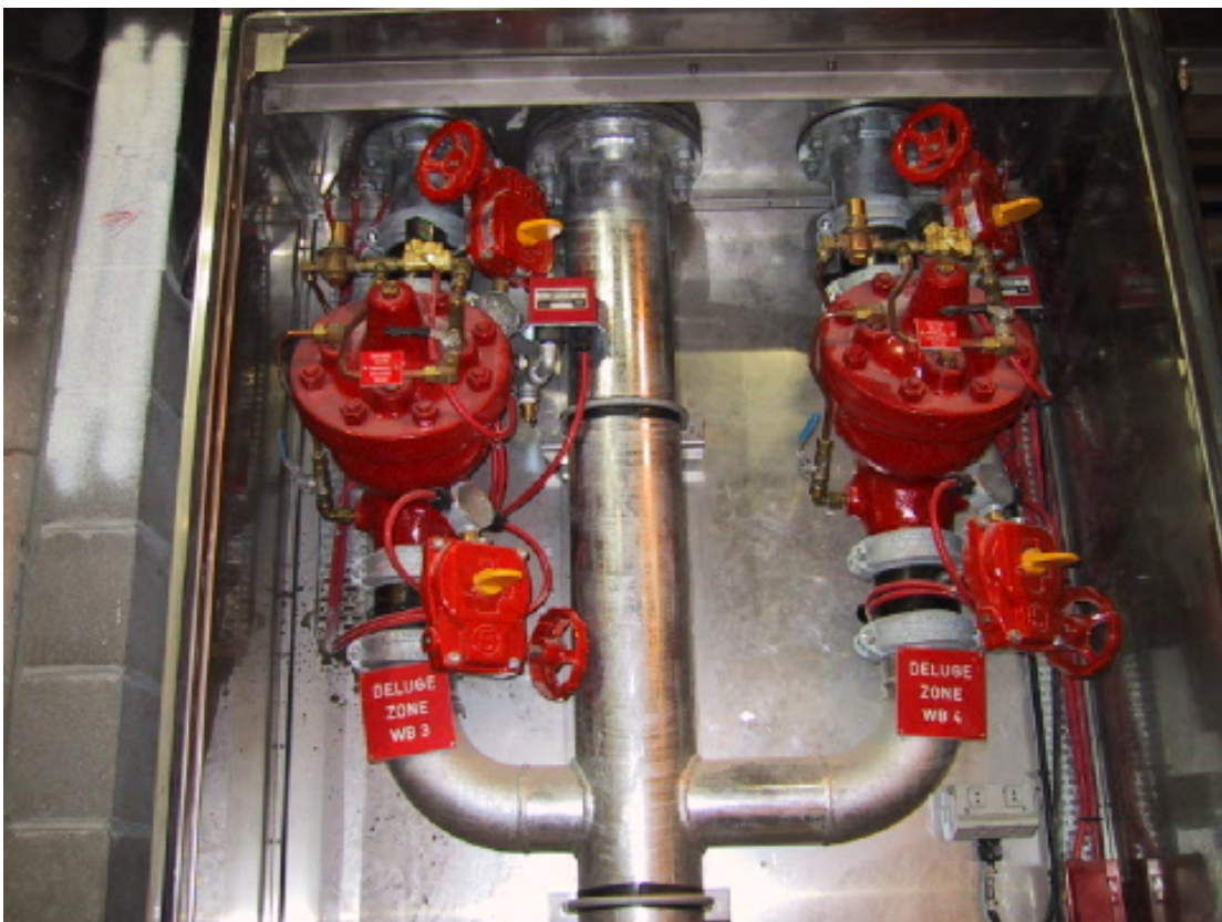
Figure 5 Drencher System Valves
