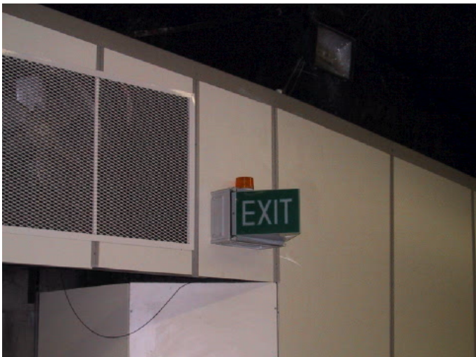
Figure 2 Exit Sign with Strobe Light
