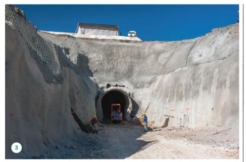
Micro tunnels are under construction in Mostar for the main sewage collector. The Contractor is Ludwig Pfeiffer Hoch-und Tiefbau GmbH & Co. The value of the works is €5.5M. The
