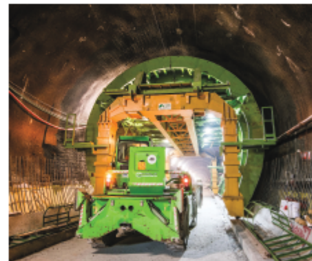
Brenner Base Tunnel: Permanent lining casting
