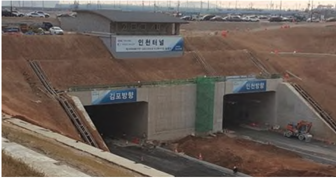
Incheon (North Port) Subsea Road Tunnel Construction
