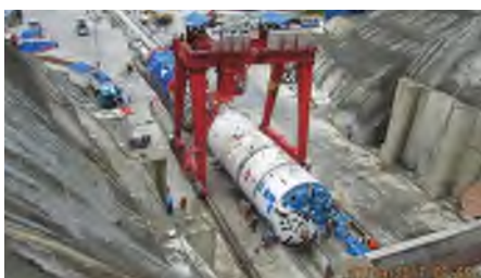
The 5.2m diameter Double shield TBM ready for excavation on the Bheri Babai Multipurpose Project
