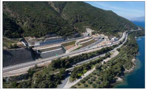
railway line, 21.5km long, between ch. 91+500 to ch.113+000. It includes the Panagopoula twin tunnels (each approximately 4.800m long).
