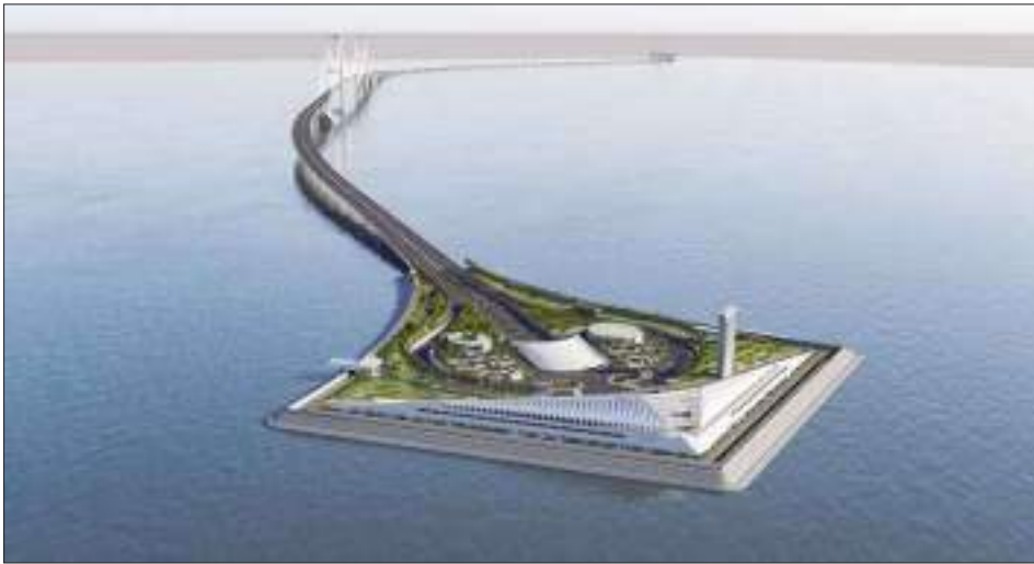
Shenzhen-Zhongshan Channel Project
