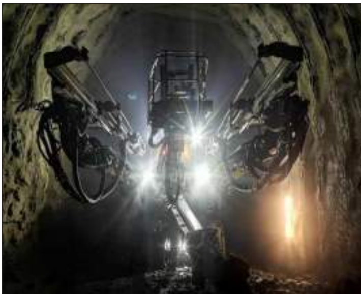
The single-track Dusse-Alinsky tunnel
