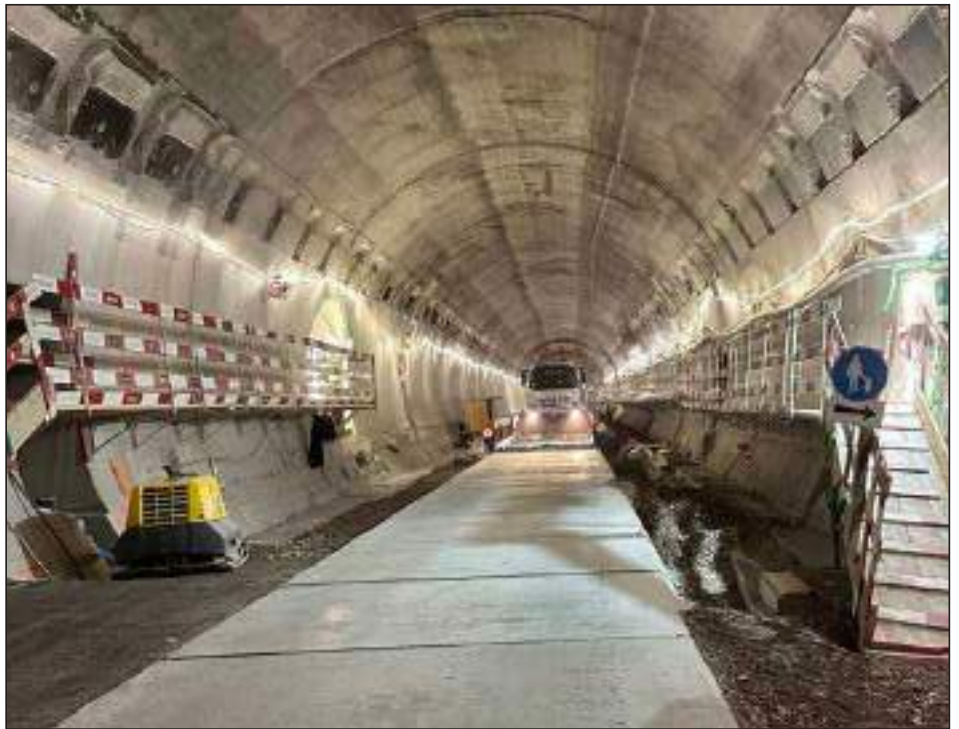
Gubrist highway tunnel 3rd tube
