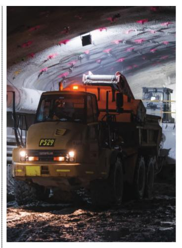
CPB/Samsung/John Holland JV is continuing with the design and construction of the A\$2.7bn M4 East project (WestConnex Stage 1B) in Sydney. The project includes twin 3 lane road tunnels, each 5.5km in length and requires 18 roadheaders to mine the tunnels through Hawkesbury Sandstone and Ashfield Shale. The project is planned for completion by 2019.
