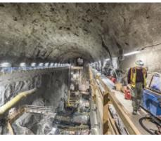
underground powerhouse, and main access tunnel had been completely excavated: 2/3 of the 1575m long power tunnel and 3/4 of the 520m long tailrace tunnel remained to be excavated. It took 13 months, 485 blasts, to excavate the 60,000 cubic metres of rock for the powerhouse cavern.
