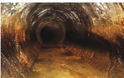
Rehabilitation of the 14km long tunnel of the Tunjita Hydroelectric Project.
