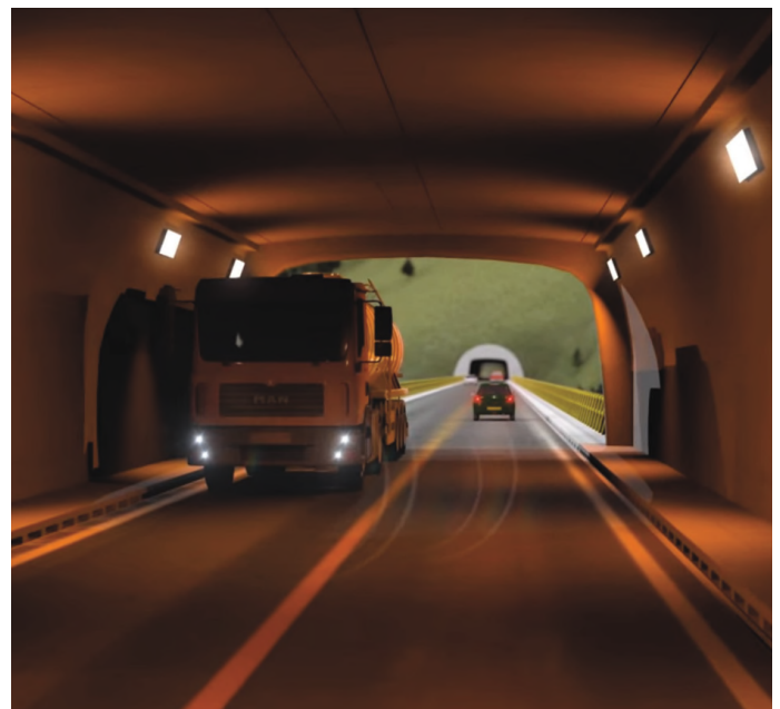
El Toyo Tunnel. Taken from Antioquia State Government
