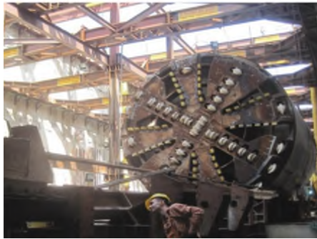
Dragging of TBM across government estate station box in progress
