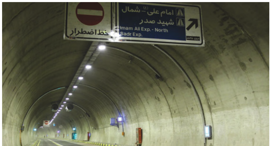
Amir Kabir Tunnel
