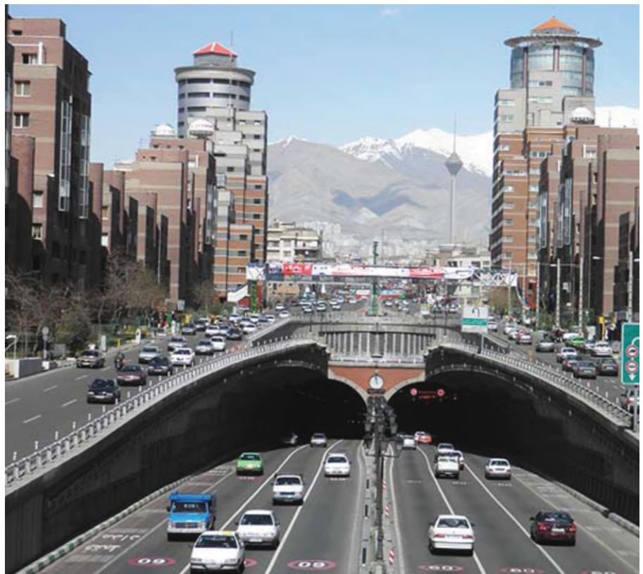
Southern portal of Touhid Tunnel
