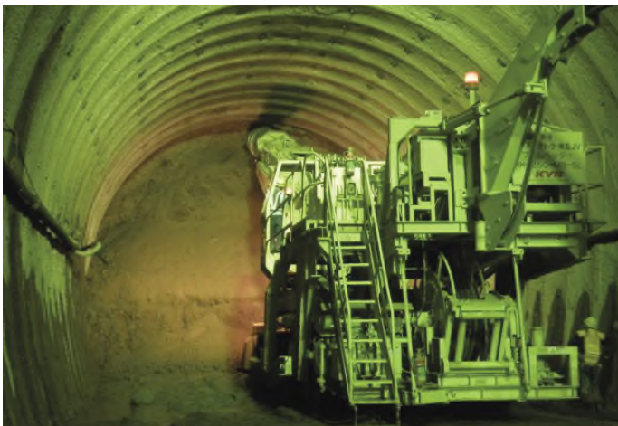
Northbound's shield: "Two independent rotating cutterhead"
