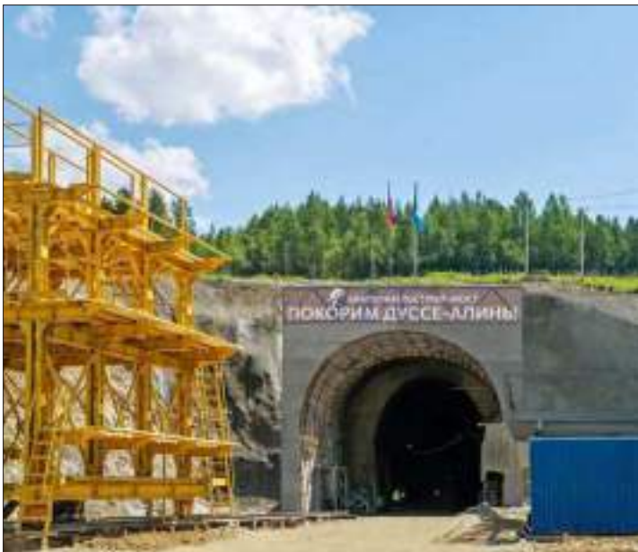
Dusse-Alinsky railway tunnel
