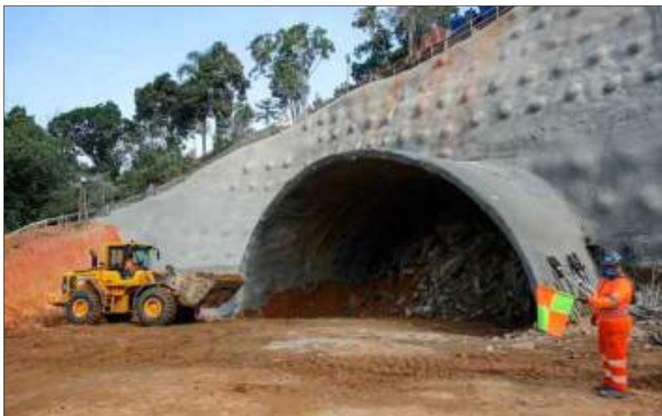
Contorno Viário de Florianópolis: Tunnel 1 begins to be excavated in Palhoça (Photo: Arteris, Disclosure)
