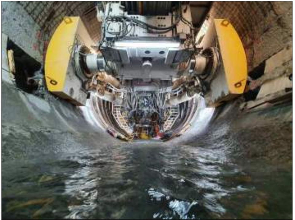
Flood protection for the Sarneraa valley
