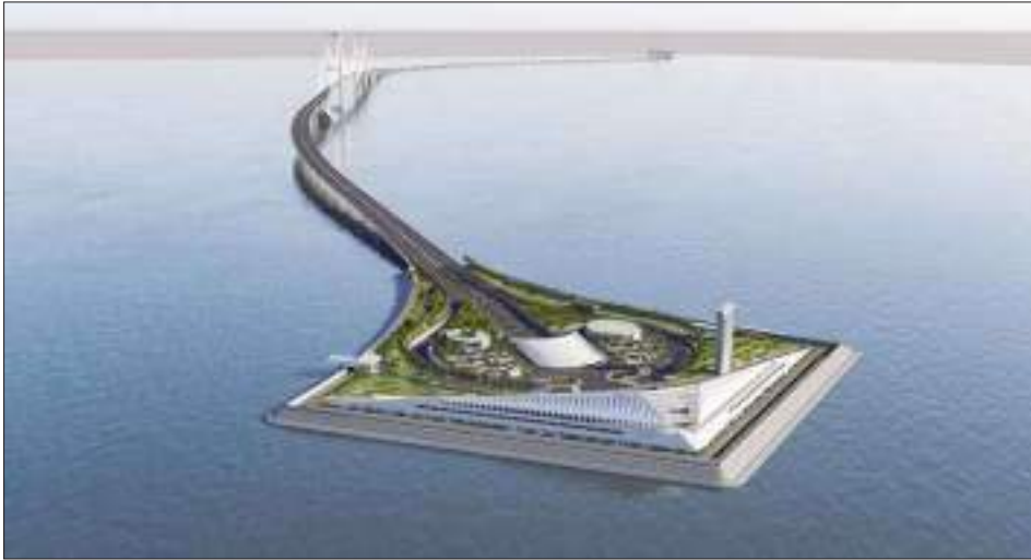
Shenzhen-Zhongshan Channel Project
