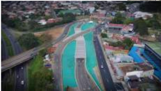
Above: La Galera Underground Pass Right: Garita Hydroelectric Tunnel
