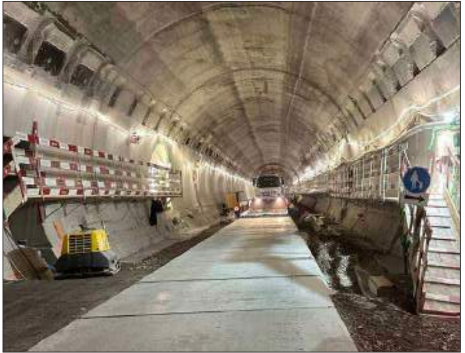
Gubrist highway tunnel 3rd tube
