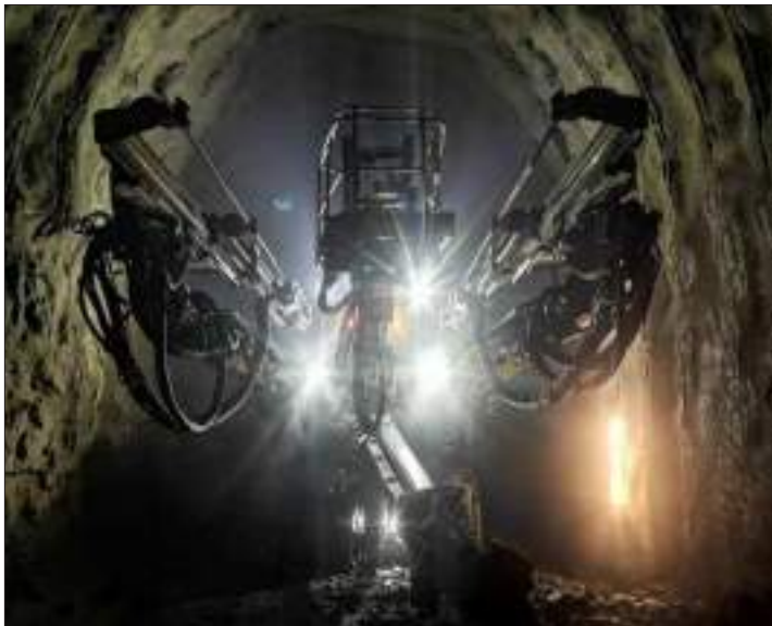
The single-track Dusse-Alinsky tunnel
