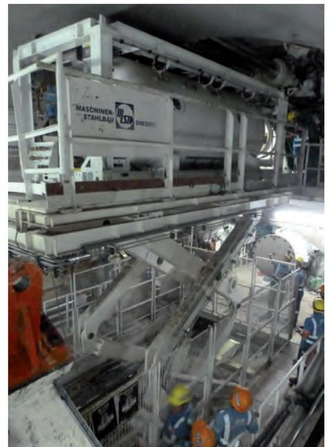
Figure 2 : TUP shuttle being mated to TBM lock
