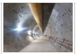
reclamation plants for further processing and treatment. With Phase 1 completed in 2008, DTSS Phase 2 comprises of 60km of link sewers (50km of which to be constructed via pipe jacking) and 40km of deep tunnels at depths between 35m to 55m, both underground and undercrossing the sea. A total of 19 TBMs, comprising of both EPBMs and Slurry TBMs, will be used to construct the deep tunnels.
