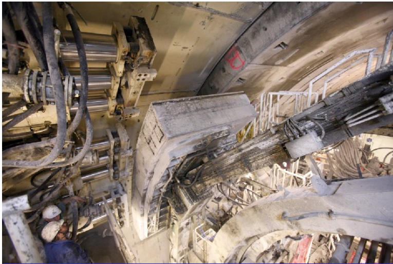
PLACING OF SEGMENTS
