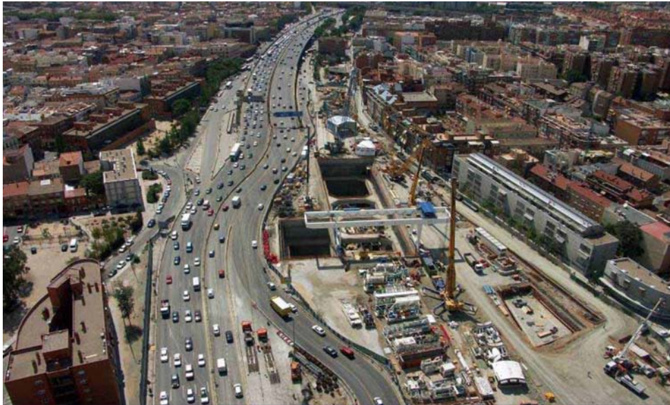
TBM LAUNCHING SHAFT – SOUTHERN BY-PASS
