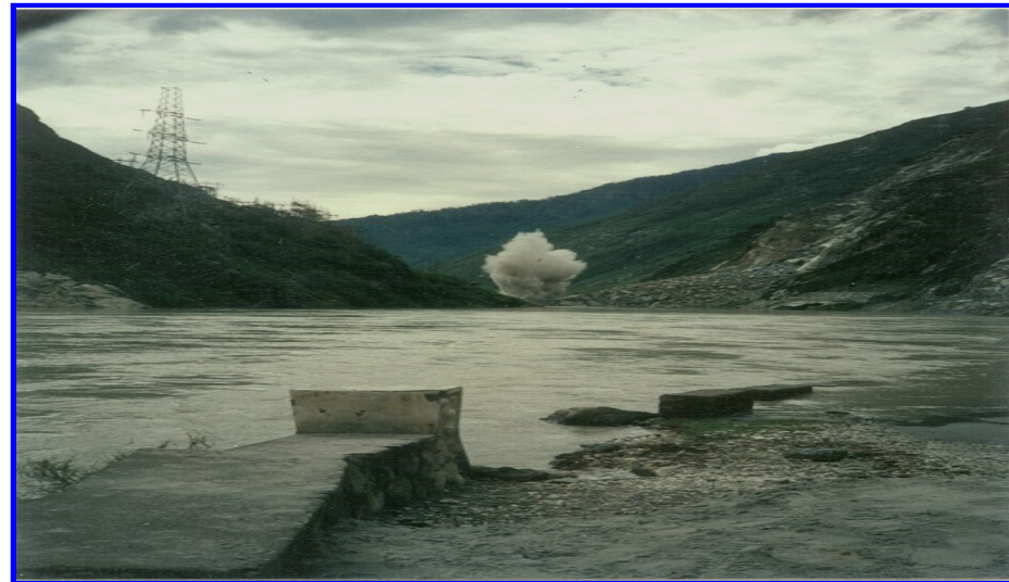
Rock slide removal by blasting
