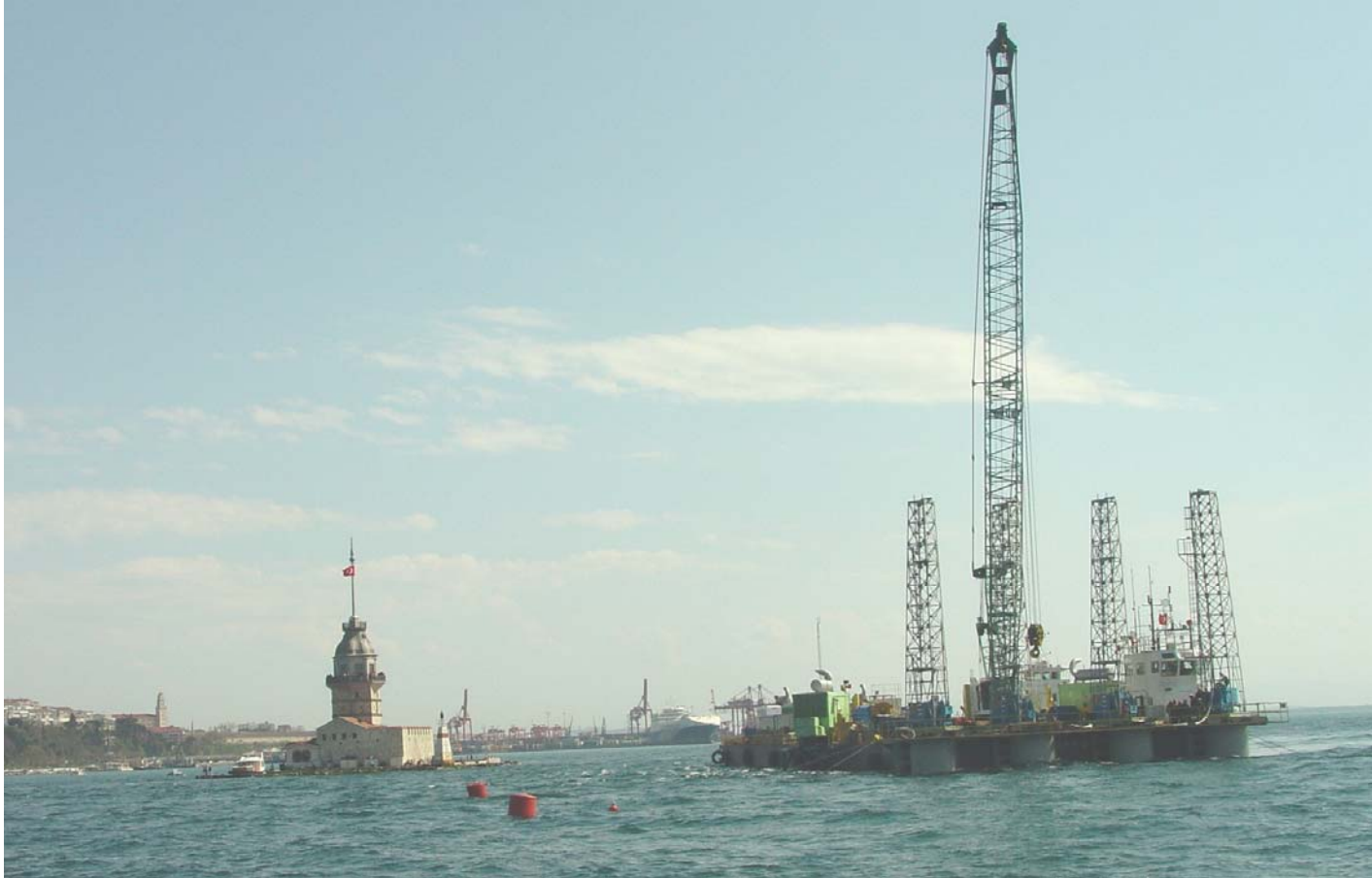
Compaction Grouting barge “SAR III”: 86 x 24 m
