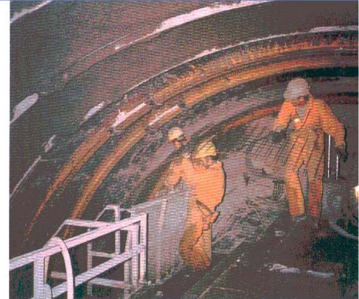
Space is available on the machine for fitting of wire-mesh support and ring beams
