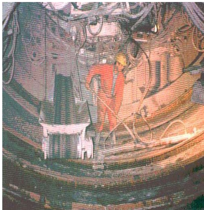
The clearance underneath the machine allows invert cleaning and transport of invert segments.
