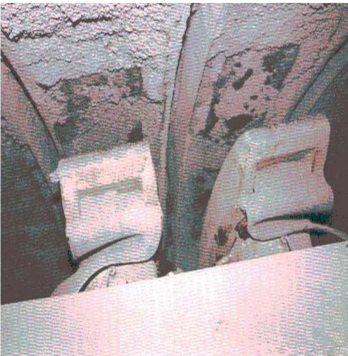
The support rings installed are bridged to avoid damage; the geometry of the grippers is tailored to this.
