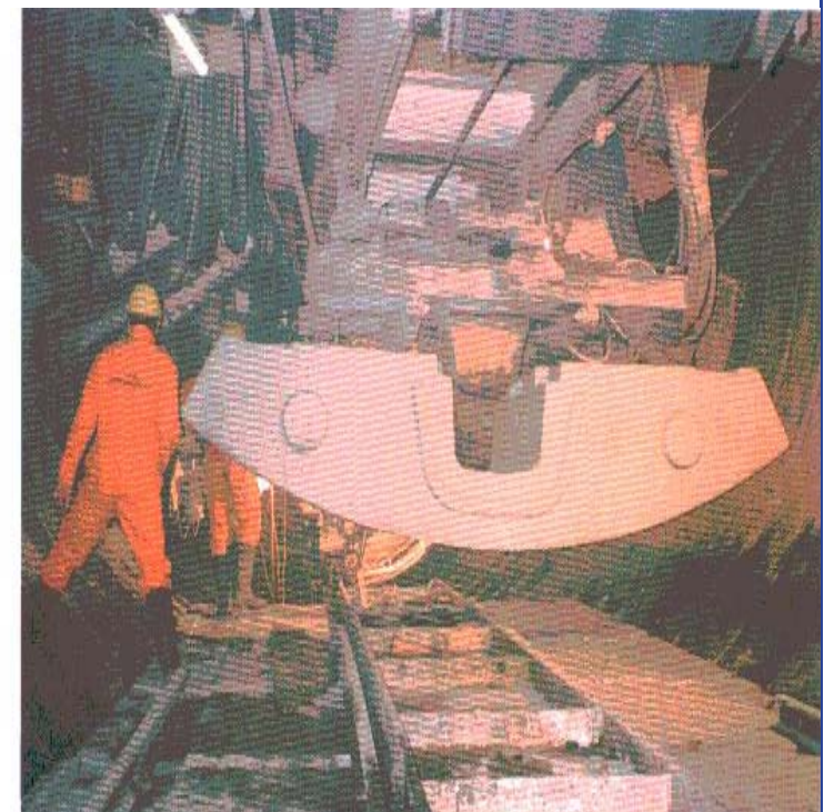
The clearance underneath the machine allows invert cleaning and transport of invert segments.
