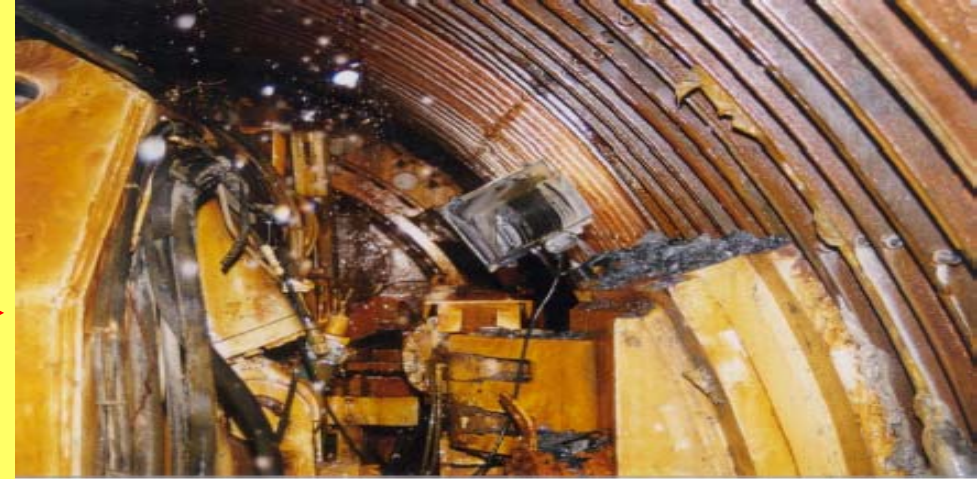
Pont Ventoux Hydroelectric Power Plant Crumbling behavior in a fault zone: heavy support behind the head of the TBM (from Barla and Pelizza, 2000)
