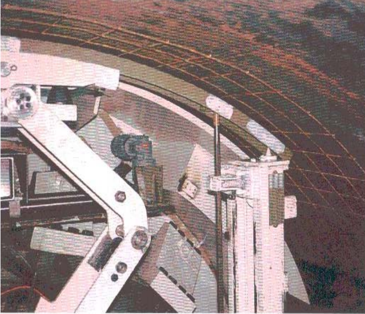
Ribs and wire-mesh support are mechanically installed directly behind the cutter head
