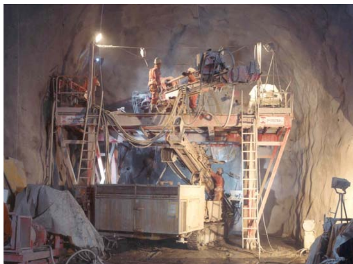
Figure 8. Drilling the boreholes at two levels
