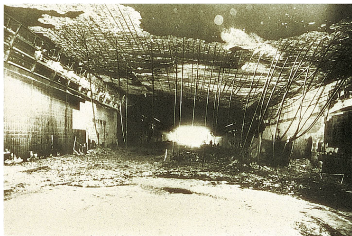
Fig. 2: Hamburg's Moorfleet Tunnel on the federal motorway following the lorry fire in 1968
