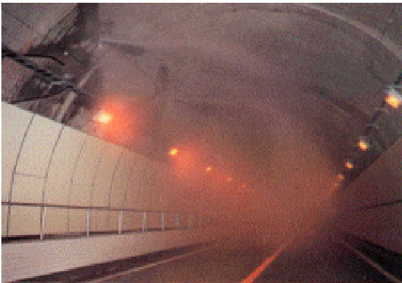
Figure 10. Water sprinkler system
