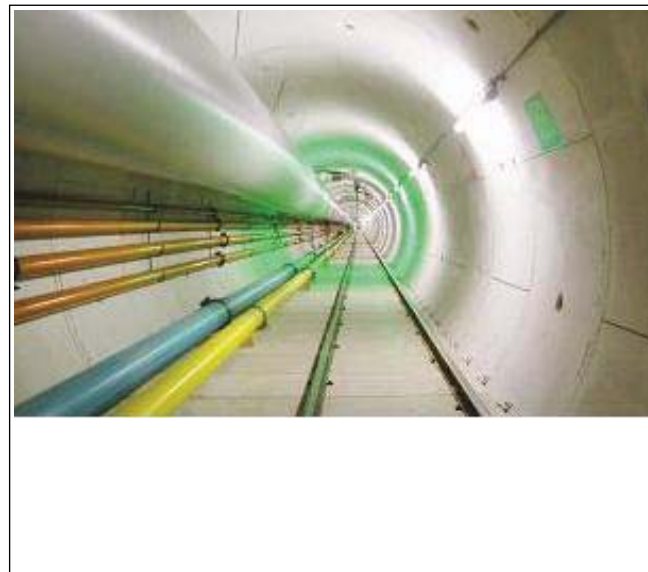
Picture 2 : Tunnel view
