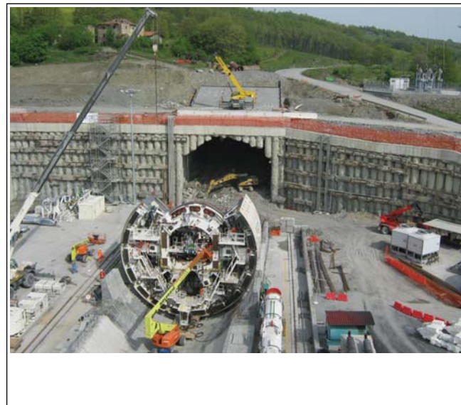
Picture 2 : TBM Assembling Area
