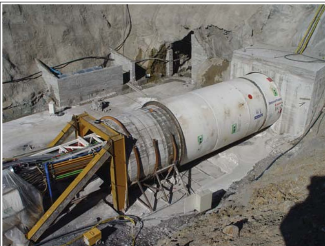
Picture 1: EPB TBM for lot 1
