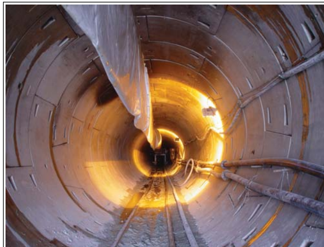
Picture 2 : lot1 tunnel lining
