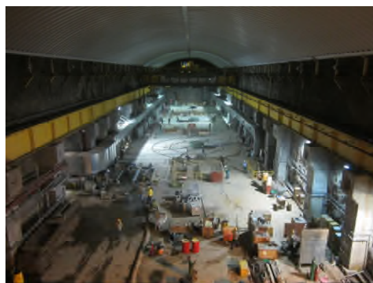
Sogamoso Hydroelectric Project – Underground cavern. Taken from INGETEC.
