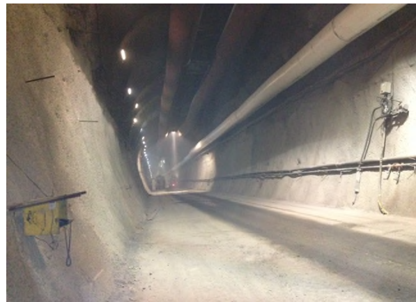
Aspect of headrace tunnel (conventional excavation), Reventazón Hydroelectric Project
