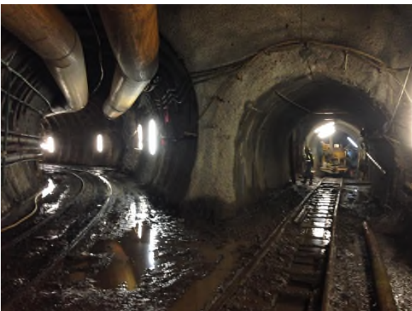
Access tunnel for Cachi Hydroelectric Project
