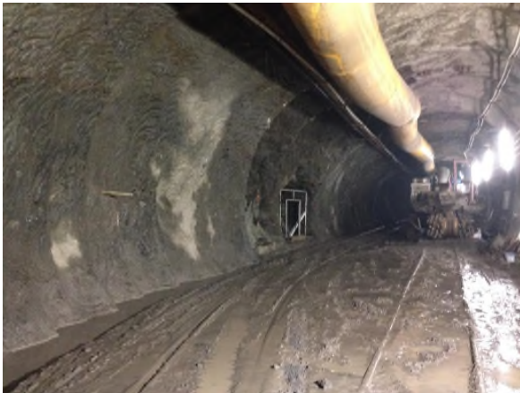
Tunnel excavated by roadheader, Cachi Hydroelectric Project
