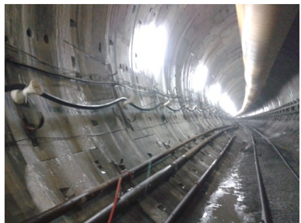
Tunnel excavated by EPB-TBM at Torito Hydroelectric Project
