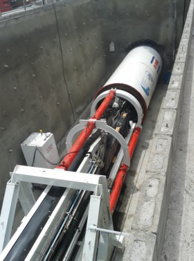
EPB ready to start excavation
