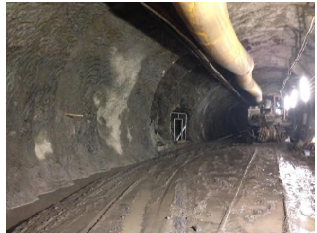
Tunnel excavated by roadheader, Cachi Hydroelectric Project
