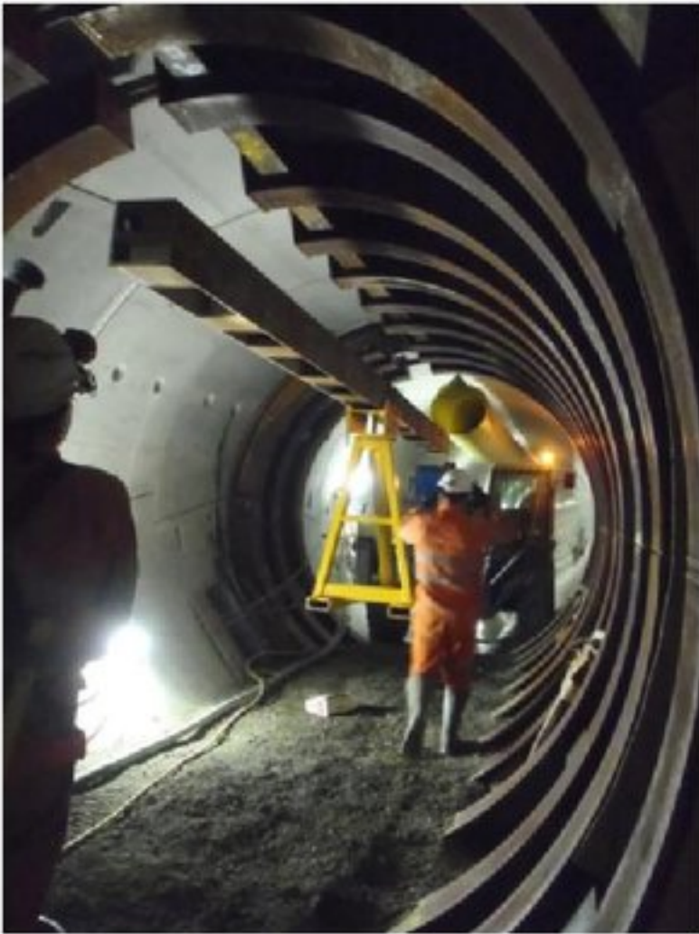
Figure 4 – Installation of Temporary Support at Adit
