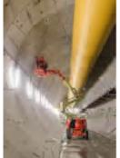
Annabell and Joyce, the Legacy Way's two tunnel boring machines, have reached the one-kilometre mark on the 4.6-kilometre tunnel, which will connect the Western Freeway at Toowong with the Inner City Bypass at Kelvin Grove. Both TBMs have set record advance rates for machines larger than 12 m in diameter. Best day of 48.9 m and average daily production of 23 m since the start of tunnelling.
