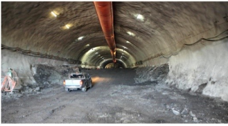
Northbound Tunnel from South: Heading and Bench Excavation
