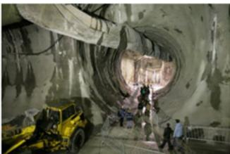
The entire length of the **Dejvice tunnel** section is 1.0 km, the whole section is cut and cover tunnel structure, this section runs under the Milady Horakove Street. Majority of tunnelling works on this section was completed from 2008 to 2010.
