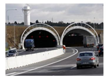
The **Komorany tunnel** (Lot 513) is 1.9 km long, its construction was done by Skanska a.s., the **Lochkov tunnel** (Lot 514) is 1.6 km long, its construction was done by Skanska a.s. Both tunnels have one double-lane tube for the descending direction and three-lane tube for the ascending direction, tubes are connected with cross-passages, excavation was done using NATM. The both tunnels were opened to
