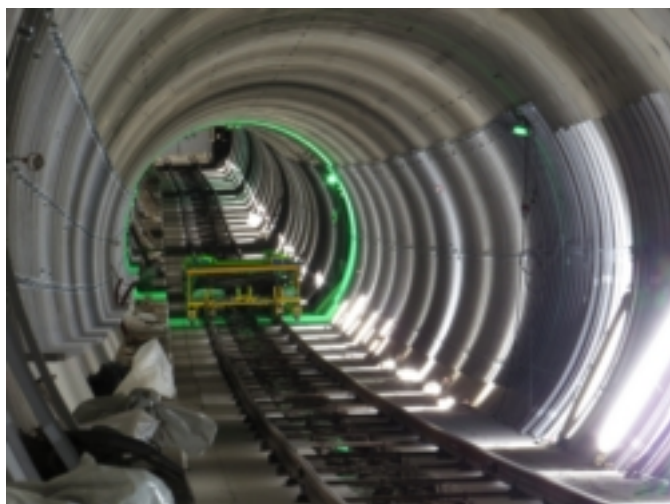
Connection of the left-hand track to the existing metro line (photo Metrostav a.s.)
