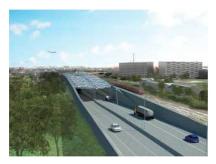
The first phase of the Marselis Boulevard Tunnel in Aarhus - connecting the Motorway system and Ring Road network with the Port of Aarhus - is under construction. The second phase with a 2 km cut & cover tunnel is delayed due to problems with the financial founding's.
