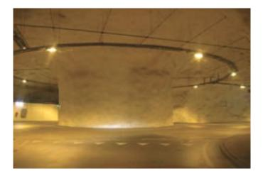
When considering rock mechanics, the most challenging section was the crossing of the crushed zone of Kluuvi area. Also the groundwater level was strictly observed by the authorities, no decline of the water level was allowed due to the tree props of some buildings in the city center. In the tunnel the first underground traffic circles have been introduced.
