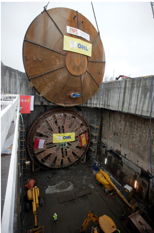
Fig. 3 Break through – tunnel under Martwa Wisła River in Gdańsk
