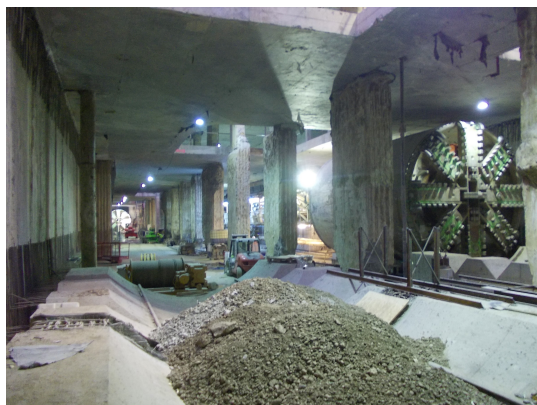
Both TBM's in Orizont Station.
