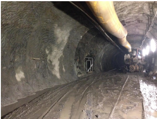
Tunnel excavated by roadheader, Cachi Hydroelectric Project
