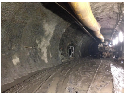
Tunnel excavated by roadheader, Cachi Hydroelectric Project
