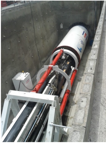
EPB ready to start excavation
