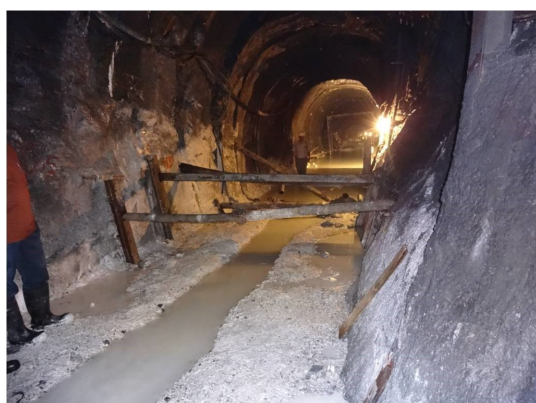
Mai Hydroelectric Project headrace tunnel lining squeezed headrace tunnel
