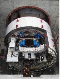
Ø10.9 m Slurry machine was used for the "Beijing to Shenyang high speed railway tunnel". A shallow overburden section has already been passed. This tunnel crosses below many high-raise buildings, airport highway and Metro line.
