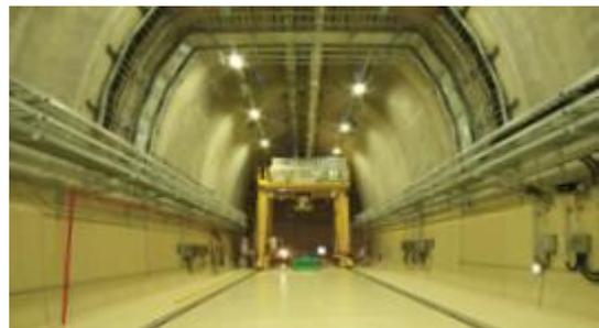
Indeed, the site can hold up to 800,000 drums (160,00m<sup>3</sup>) of low and intermediate level of radioactive waste. A disposal facility was constructed to store 100,000 drums (20,000m<sup>3</sup>) of LILW. It consists in six silos storing LILW and a 3.9km access tunnel.
