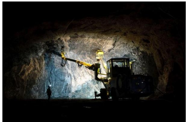
connecting tunnels and areas for technical equipment. Conventional drill and blast method with top modern equipment were used. The total rock volume is 320 000 cubic meters and the total length of the tunnels and caverns is 3000 meters. The scope of the project led to the division into two contracts:
